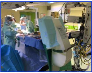
The Sterile Air Flow units enable upgrading an existing ISO 7 operating theatre to ISO 5 or extending the sterile zone in an existing operating theatre in order to prepare the instruments and implants under sterile conditions and to guarantee the best aseptic conditions during the operation.
