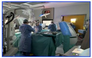
In spine surgery two mobile laminar air flow units are often used to protect both the instruments and the operating area. This technology can be used in any existing operating rooms without costly reconstruction work. This laminar air flow is perceived by the staff as very pleasant, as it does not generate cold air.
