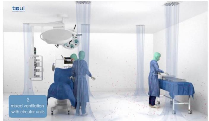
**Air filtered through conventional ventilation systems is first directed towards the floor and then distributed homogeneously throughout the operating theatre. Despite all measure to maintain asepsis, the floor of the operating theatre is always contaminated. Thus bacteria can be transmitted to the patient through the instruments and surgical wound.**
